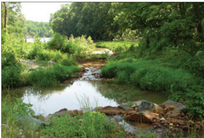
Figure 5. Riffle-weir restoration in Anne Arundel County, MD. The creation of low-velocity environments, such as step pools, increases hydraulic retention and contact time with the benthos, potentially leading to increased N removal in the channel.
