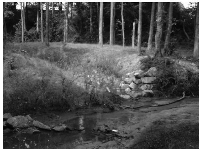
Fig. 2 Photograph showing a representative restored stream, located in northern Anne Arundel County, Maryland. Large boulders have been placed on the channel banks to prevent bank erosion and have been placed in the channel to prevent channel incision.
